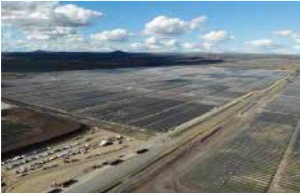
Location: Australia Capacity: 134MW Technology: Arctracker Pro
