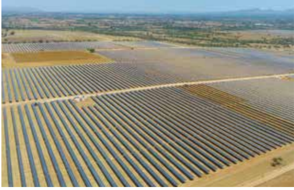
Location: Mexico Capacity: 118MW Technology: SkyLine Tracking System + Bifacial Modules
