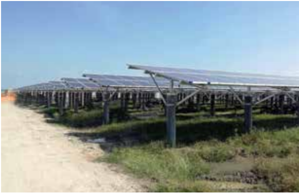
Location: Vietnam Capacity: 500MW Technology: Fixed Structure
