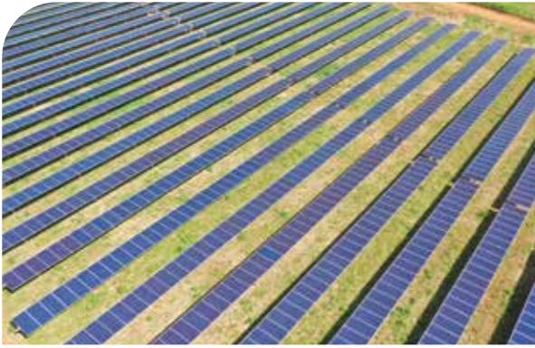
Location: Malawi Capacity: 75MW Technology: SkyLine Tracking System
