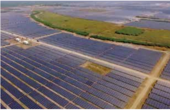
Location: India Capacity: 648MW Technology: Fixed Structure
